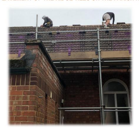
At the beginning of this month, we replaced the ridge tiles on the parish hall. They were loose and in very poor condition and there were several cracked roof tiles which were also replaced.
